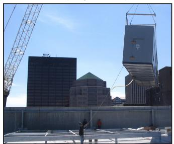
The first of 14 sections of a rooftop unit for the CareSource project is put into place by the Rieck Services' construction team.
